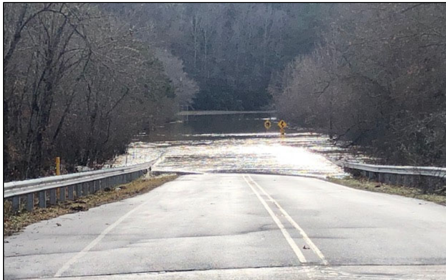
Exhibit 2. Wilson Road closure at the bridge abutment (facing south) due to flooding December 2018 (NCDOT).
