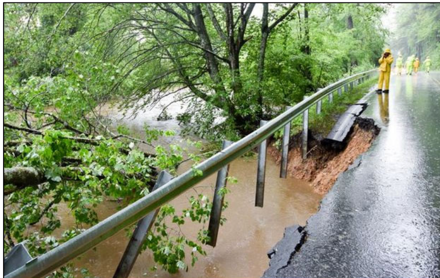
Exhibit 3. Wilson Road, between US 276 and Elm Bend Road, collapses after heavy rains May 2018 ( Transylvania Times ).
